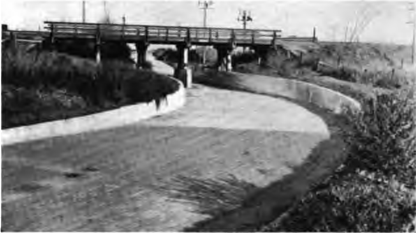
San Joaquin County's highways are built for safety. Subway on Borden Highway protected from seepage by concrete walls.
